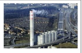
used to produce steam that spins a turbine (a steam wheel) and hence generates electricity. The remaining heat from the process can be used to heat buildings of the neighboring area. In many cases, the primary goal is to produce heat rather than electricity.
