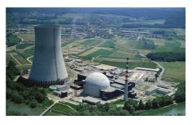
The remaining heat from the process can be used to heat buildings of the neighboring area. If there are no heat consumers nearby, the steam cycle is cooled down by using river or lake water or is cooled down in cooling towers, using an additional water cycle.
