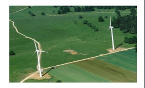
can shift direction in order to generate most electricity at every direction and speed of the wind. In case of storms, the plant automatically stops and twists its blades not to catch wind. Wind power plants can be built as stand-alone plants or as parks with multiple plants.
