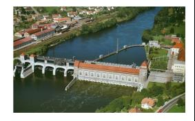
accumulate water and thus rely on the natural flow of the river. Some run-of-river plants can include a dam that extends to a part or the full width of the river in order to aid water flow regulation. But the dam's effect on the water level in the river is minimal.
